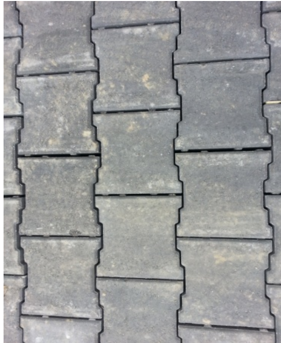
Figure 28: PaveDrain pavers in Louisville's CSO130 installation
