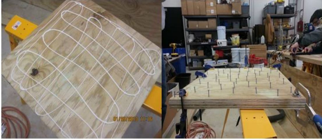
Figure 12: Construction of the flume's panels
